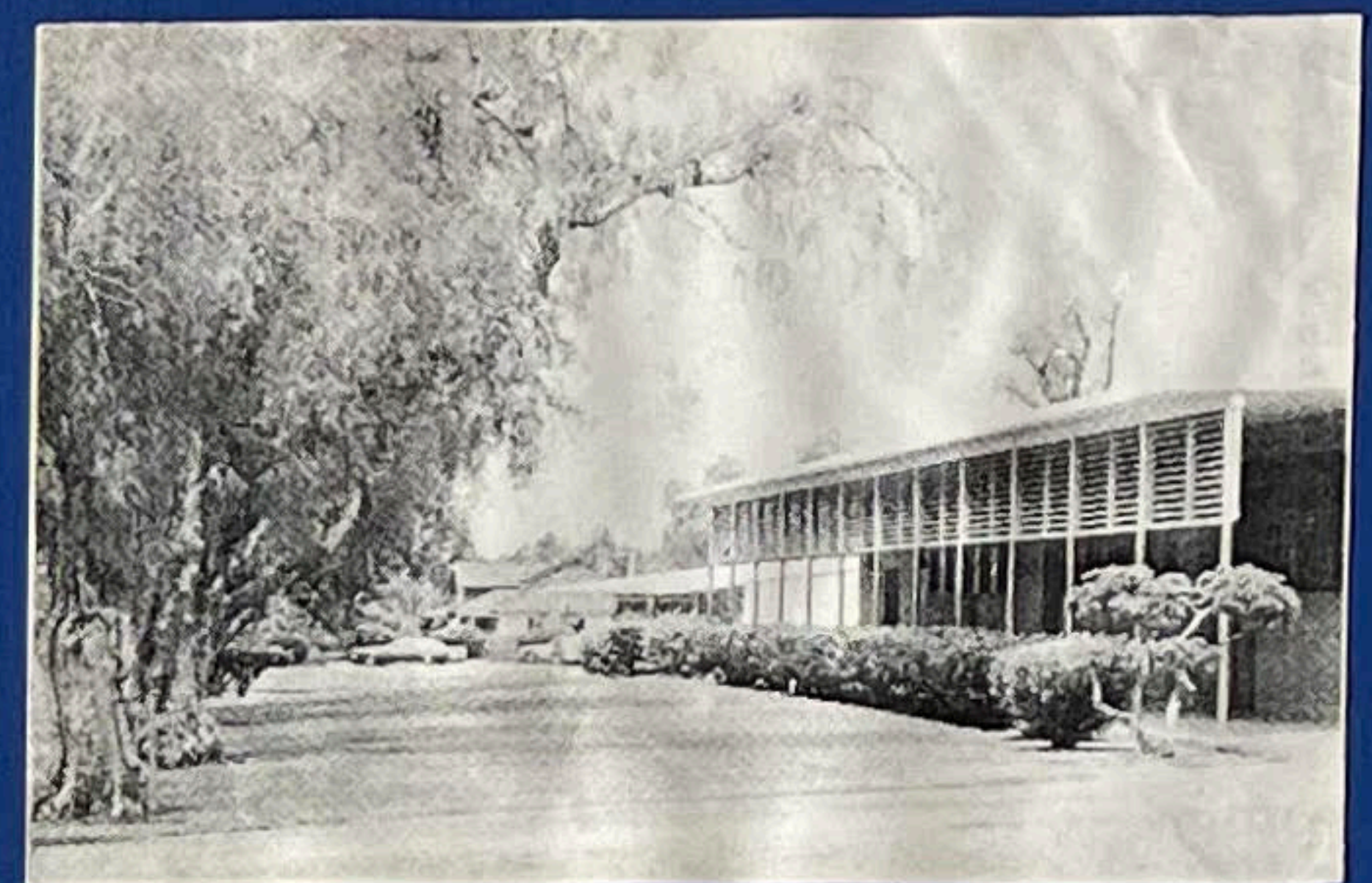
This building, constructed in 1926, is used for storage and offices at Villa Park Elementary School.
